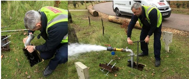
3. Fit Standpipe. (Ensure the gasket is in place at the base), and tighten.
